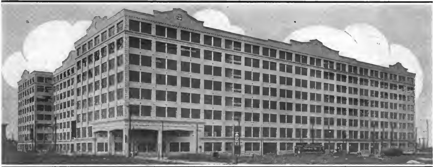
Specimen of steel reinforced concrete factory building at Bush Terminal. Tenant may have 140,000 square feet of space on one floor of this building
